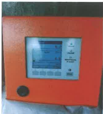
Sick Opacity meter in all stacks
