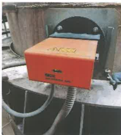
Sick Opacity meter in all stacks
